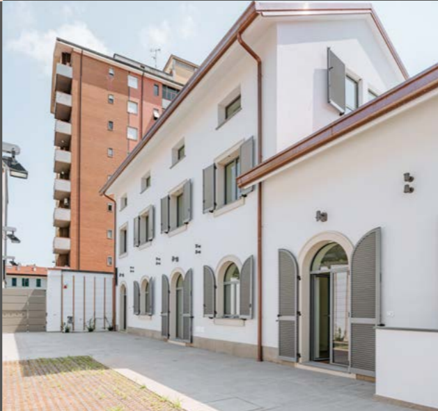
2019 - Residential building in via Alzaia (MI)
