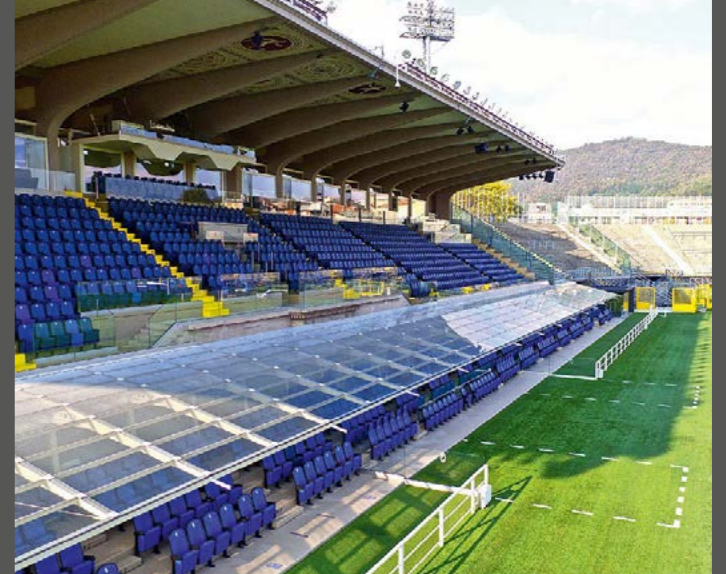
2015 - Refurbishing of the Atalanta stadium grandstand (BG)
