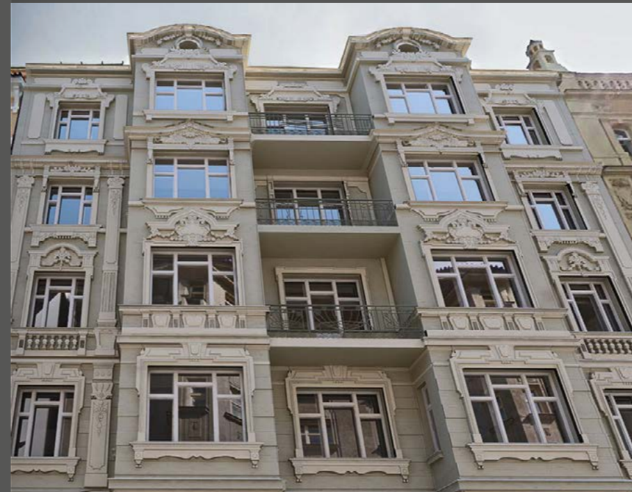
2016 - Residential building in Prague (CZ)
