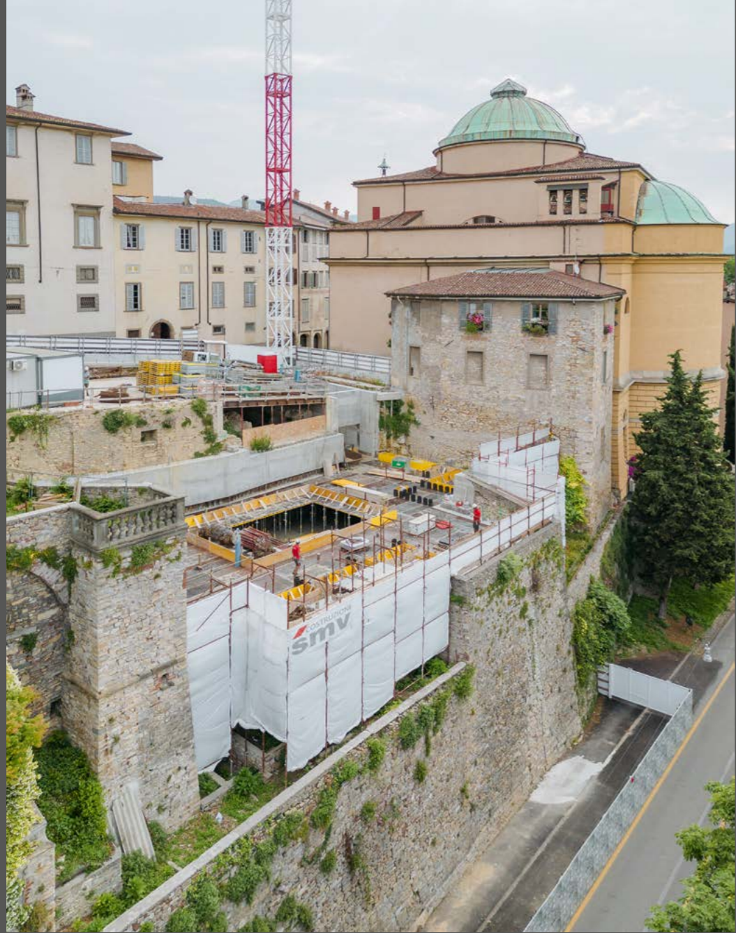
2022 - New underground garage in via Porta Dipinta, Citta Alta (BG)
